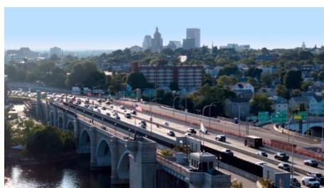
The bridge monitoring system at the Washington Bridge in Providence, Rhode Island consists of accelerometers, strain gauges, temperature sensors, inclinometers and a meteorology station – to measure, collect and interpret bridge health data, and a Weigh In Motion system to monitor specific load conditions.
