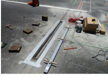
Installation of Lineas sensors from Kistler for Weigh In Motion (WIM): dynamic axle load measurement in moving traffic enables efficient bridge protection.
