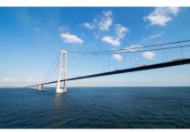
Structural health monitoring with Kistler: the Great Belt Bridge in Denmark is monitored continuously for structural changes with the aid of K-Beam accelerometers.
