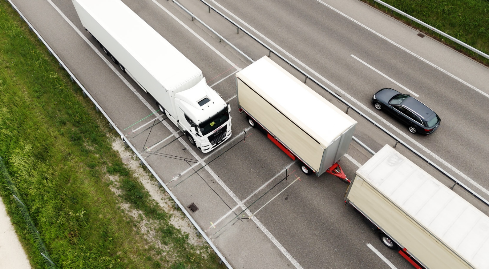
The KiTraffic Digital Weigh In Motion (WIM) system: innovative Lineas sensors are installed directly in the road surface to allow accurate measurements at speeds from 10 to 130 km/h.
