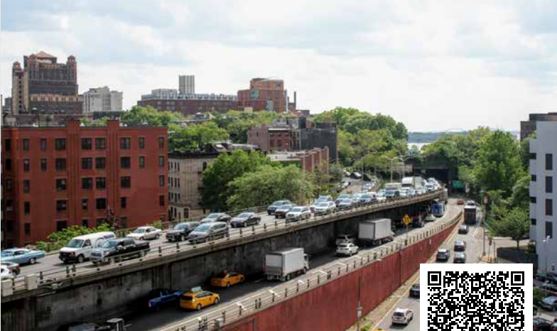
Brooklyn-Queens Expressway (BQE) built more than 70 years ago with a triple-cantilever design, 2.4km long
