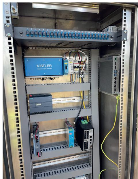
All Kistler Weigh In Motion components come prewired on a DIN rail for easy installation in the roadside cabinets for CCLEX, which are connected to the traffic management system from Indra.
