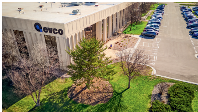
With support from Kistler sensors and systems, leading US-based manufacturer EVCO takes plastics processing to the next level for many industries including the medtech sector.
