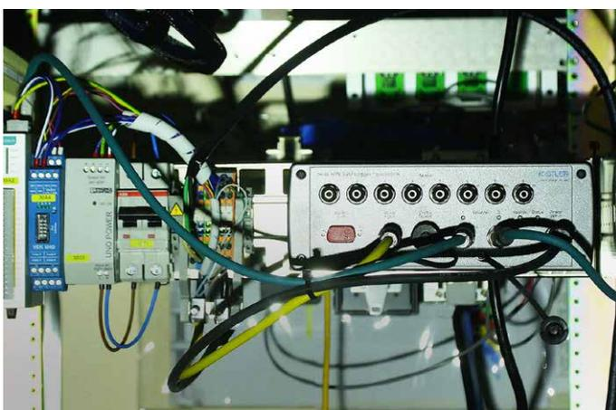
The Kistler Data Logger is installed at the road site to collect and process data, which is then transmitted to the control center and displayed in a user-friendly interface for evaluation.
