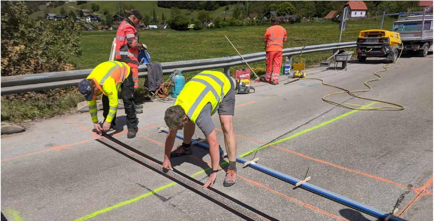
Bridge monitoring by REVOTEC on behalf of Austrian Federal Railways: installing two rows of Lineas sensors for KiTraffic Statistics.
