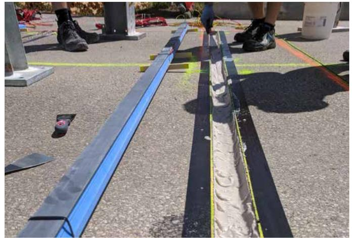
The Lineas sensors for the KiTraffic Statistics WIM system by Kistler are installed slightly below the road surface; they are coated with a special grouting compound to ensure longer lifetimes.
