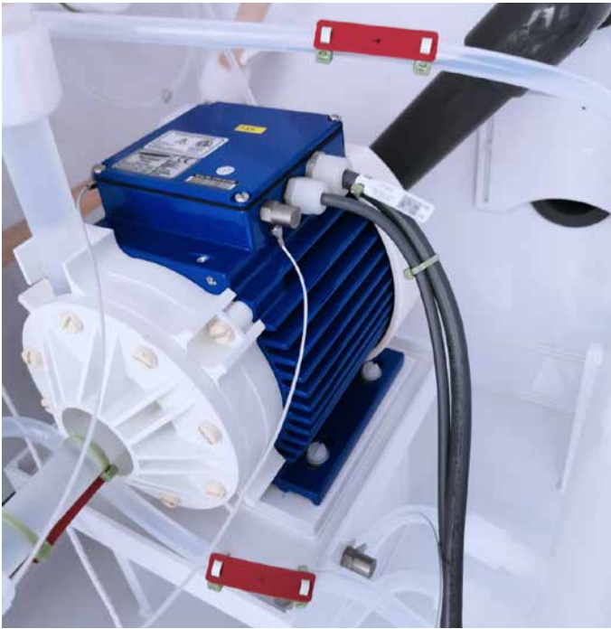
Listening in to the plant: accelerometers from Kistler examine critical components such as this chemical module pump to identify structure-borne sound patterns.
