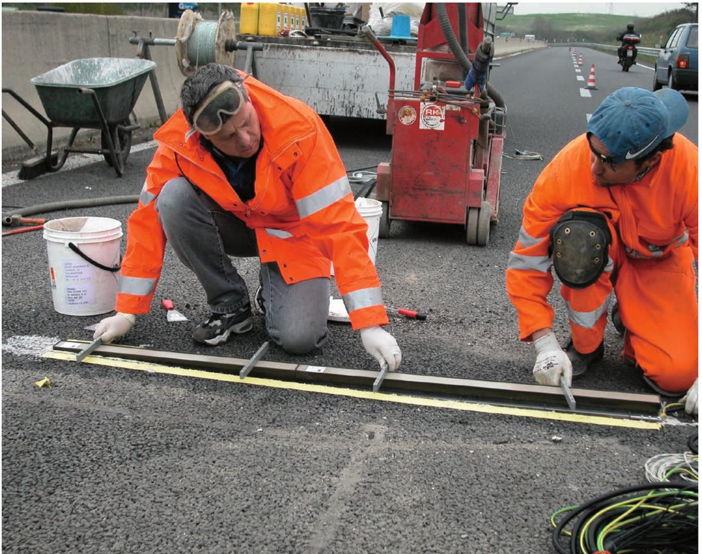
Installation of a Lineas WIM sensor.
